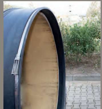
3. Position Rubber Gasket with end-clamps on bigger pipe.
