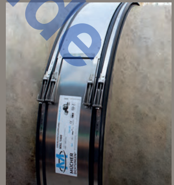
6. Tighten the bolts on the shear band evenly on each side.
