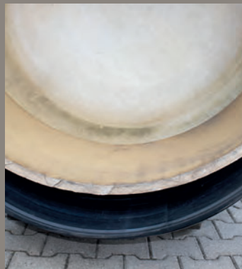
5. The bagging underneath the pipe will disappear as the clamps start to tighten.
